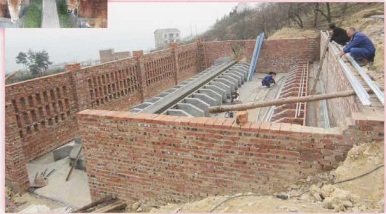
A cattle barn under construction
