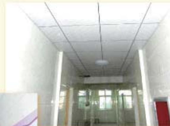
Ceilings and corridors after renovation
