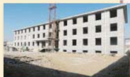
New kindergarten under construction
