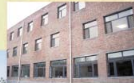
The 3-storey multi-function building
