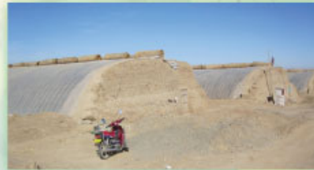
Construction of greenhouses
