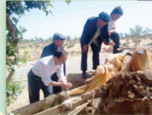
Well drilling at the site
