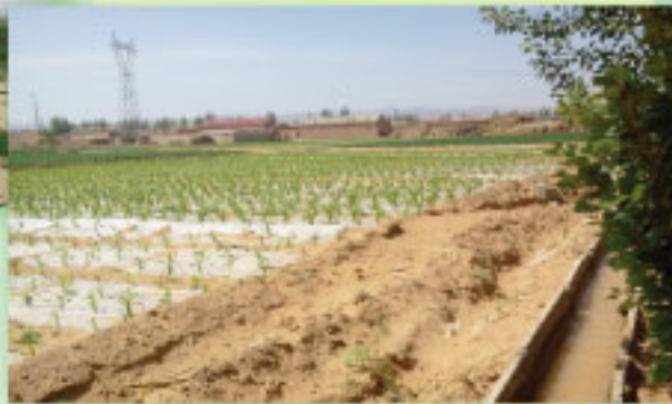
A drainage system built for irrigation of fields
