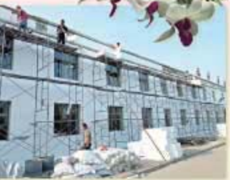
Adding Insulation to the walls
