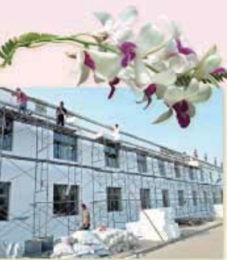
Adding Insulation to the walls
