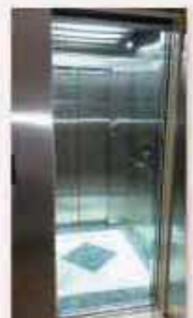
The newly installed elevator
