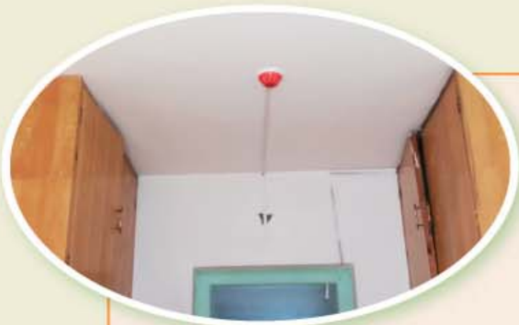
A smoke detector on the ceiling
