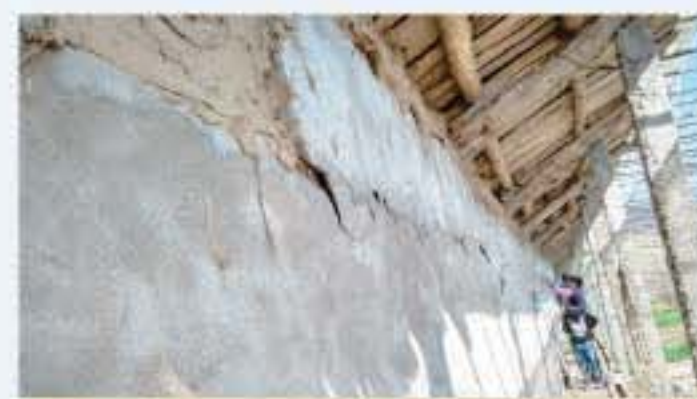
A greenhouse beyond repair
